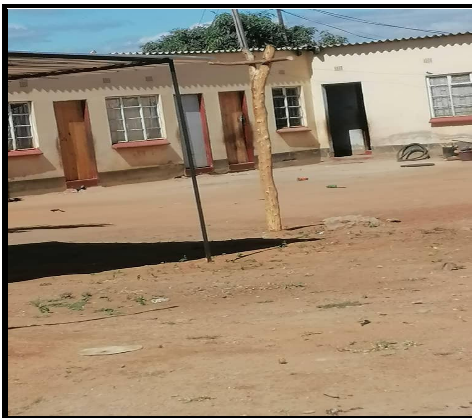
Image 5.7 Informal structures at the Zunde Home Industries in Mbizo
